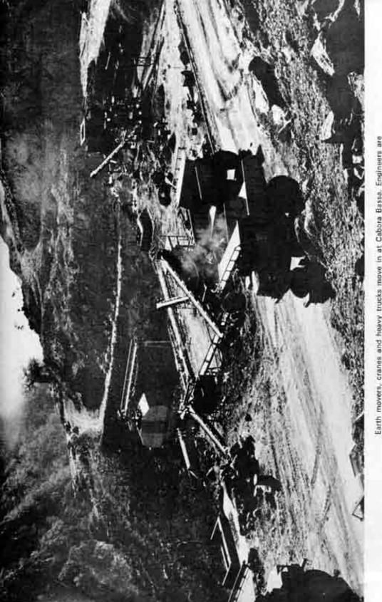
Earth movers, cranes and heavy trucks move in at Cabbra Bassa. Engineers are blassing a platform for the huge transformer station.
