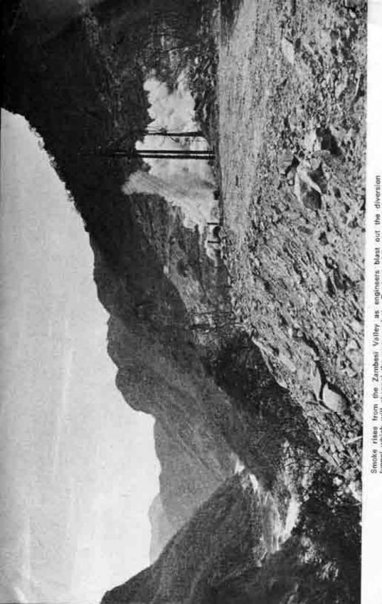
Smoke rises from the Zambesi Valley as engineers blast out the diversion tunnel which will channel the waters of the Zambesi while the dam is being built.
